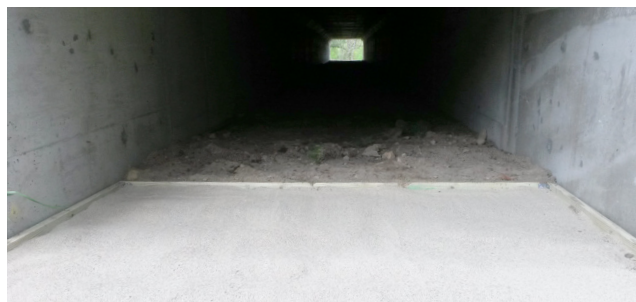
A view looking south through the tunnel from the north track bed.
