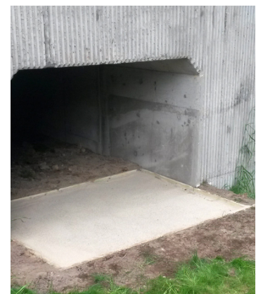
View of the south tunnel entrance and track bed.
