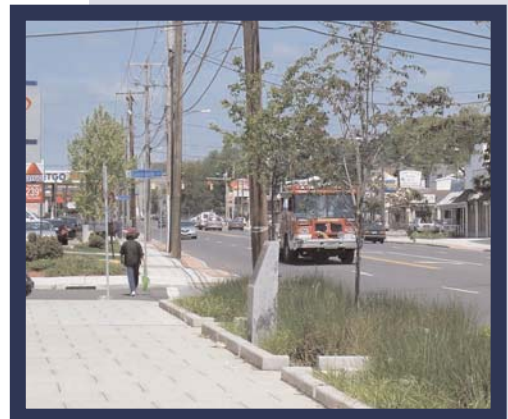
BSC created a series of rain garden bays for stormwater treatment as part of the streetscape design for Main Street in Bridgeport, CT
