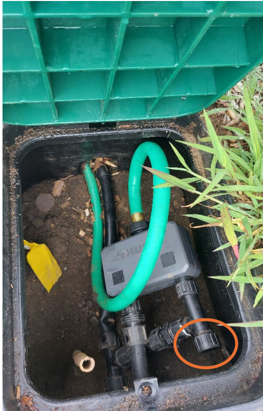
Figure 4: Vault and Controller with Filter
